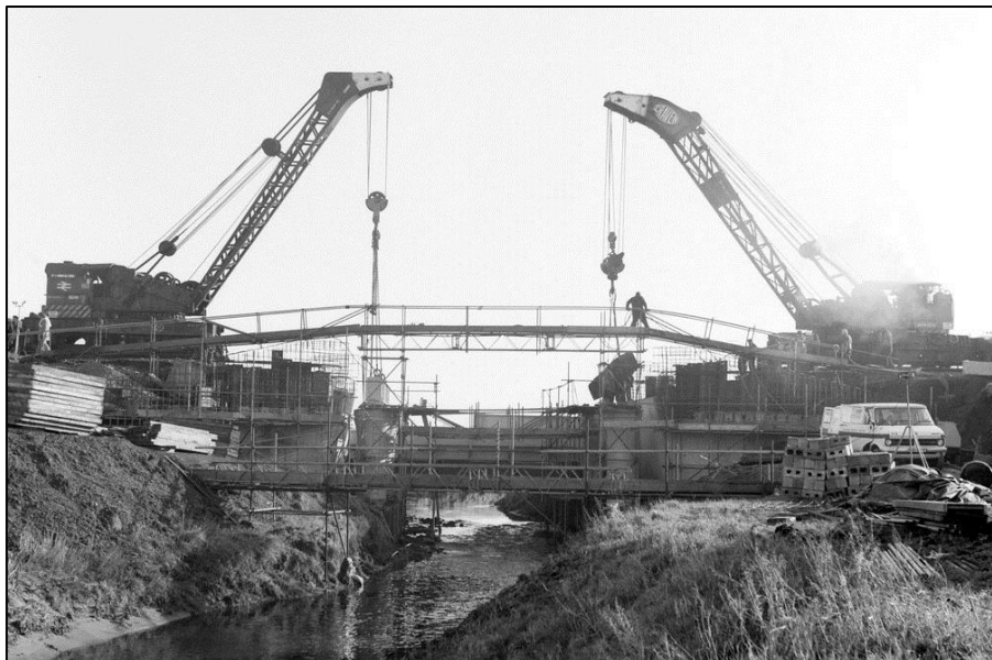
In this view looking south the two steam cranes at seen at work on the replacement of bridge No. 18 on Sunday 13 January 1980. Photo by Tony Foster
