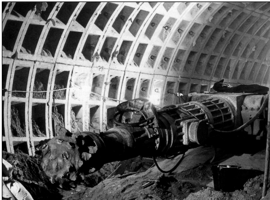
A rock drilling machine at work on the link line construction in the mid-1970s. Photo from Merseytravel
